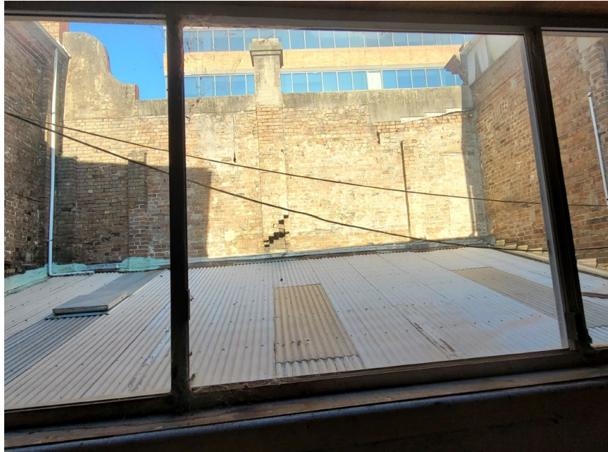
View of the parapet looking south-east towards Waterloo Street
